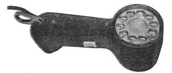
The principal application of these sets is for originating test calls on dial system apparatus for testing the switching, continuity, and talking features of the circuit. In the maintenance of the equipment, they may also be used for locating trouble in the various portions of the circuit.
