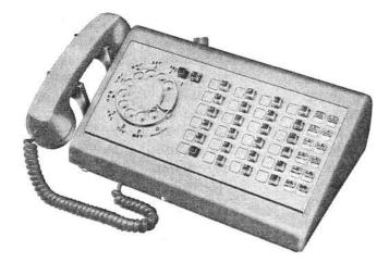
All purpose, jack equipped, large capacity five-position key telephone set with overall dimensions of 15.125 inches wide by 8.125 inches deep by 4.226 inches high. It weighs 16 pounds.
